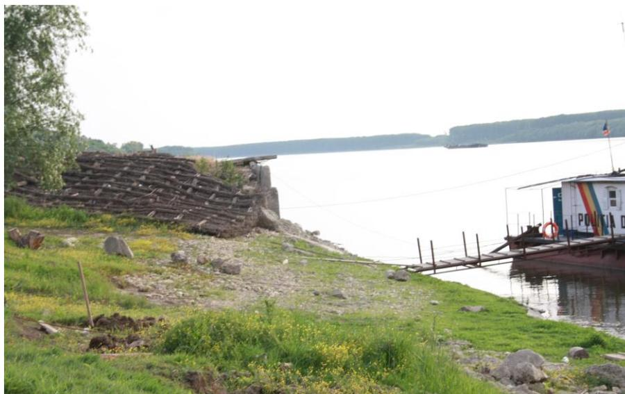
*Figure 3.1.I.7 - Fascine mattresses temporarily stored for the purpose of water transport to another location*
