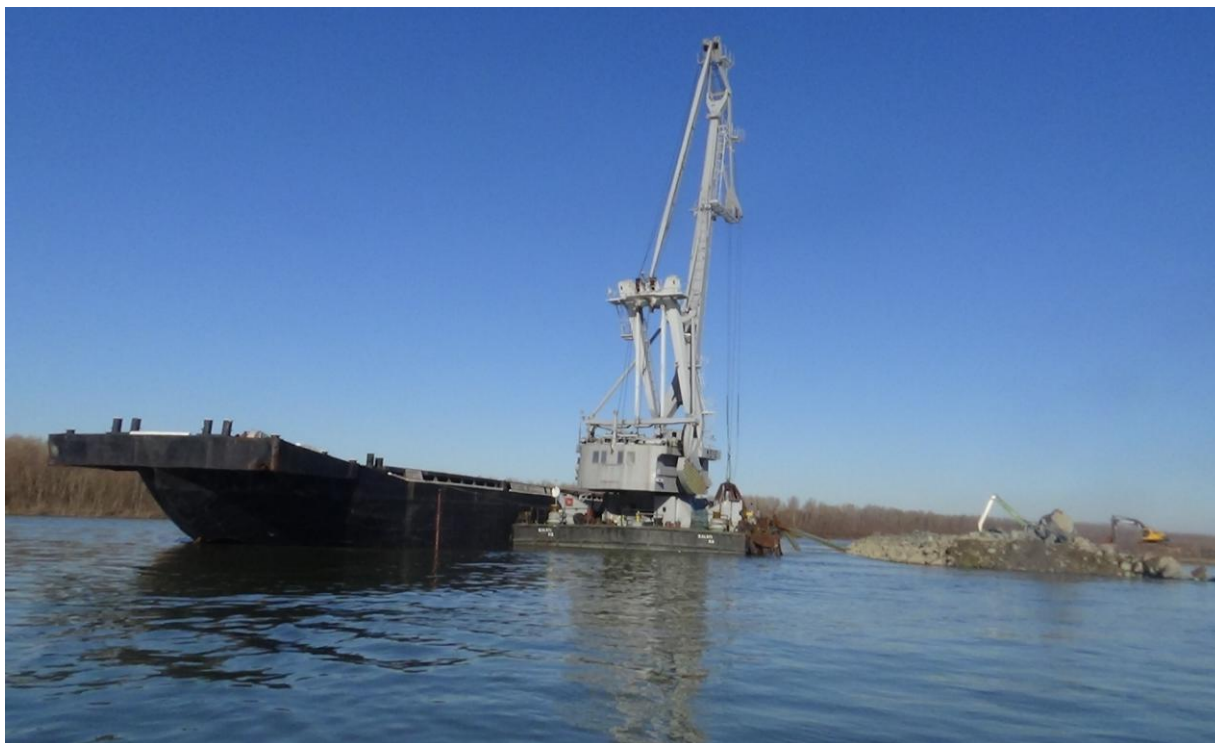
Fig.2.1.2. -Epușu PC02 - Macara, barje, excavator - mal drept
